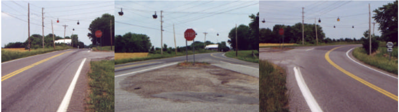
Figure V-9. Three Views of Blandville Road (US 62) at KY 286
