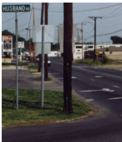
Figure V-13. Small Turning Radius And Damaged Signal Pole Close to Intersection
