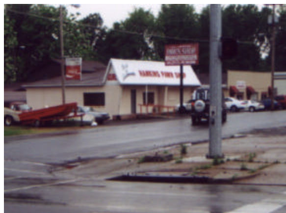
Figure V-17. Short Turning Radius on the Northwest Corner of US 45 And KY 305
