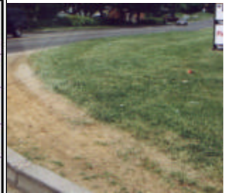
6. Improve Turning Radii for Bleich Road (KY 3074) at Lone Oak Road (US 45)
